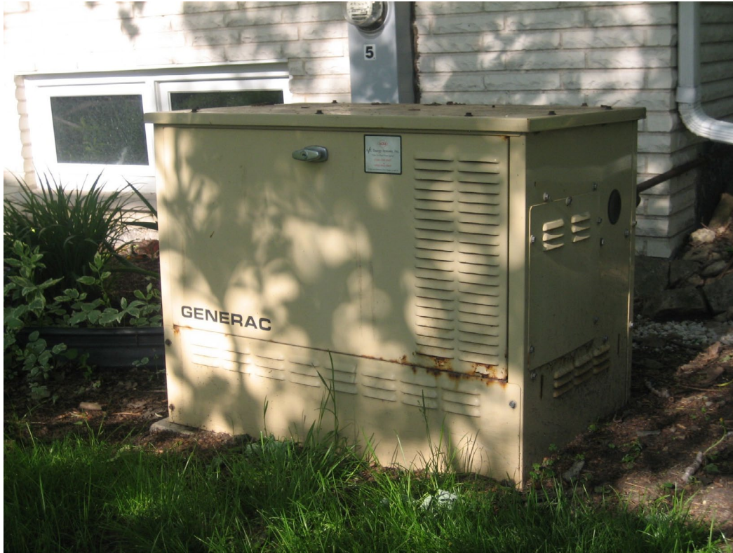
Figure 5 — A Generac 8 kVA natural gas-fired standby generator is the only source for backup power. Its weekly exercising is monitored by the BASremote.
