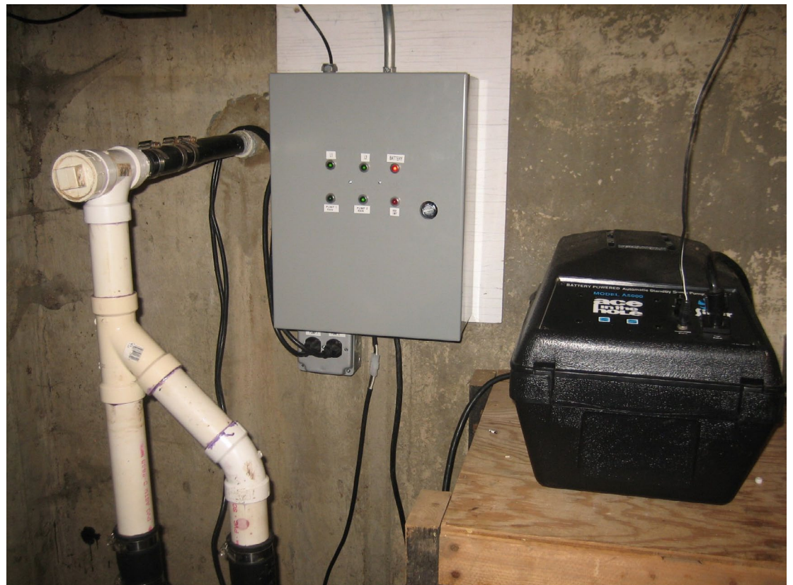
Figure 8 — Wall-mounted sump pump panel with battery case nearby. Pumps plug into a duplex receptacle alternately switched by interposing relays. An Ethernet connection is made to the homeowner's residential gateway.
